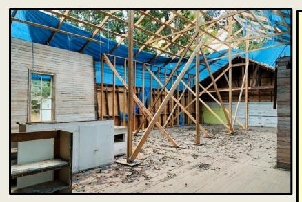
Photo is taken before the contractors began the new phase October 13. Contractor has told us the floor is in excellent condition and will be same as always with more history in its grain. Two pieces are warped in a spot, but they have assured us that they can be returned to normal with some pressure.
